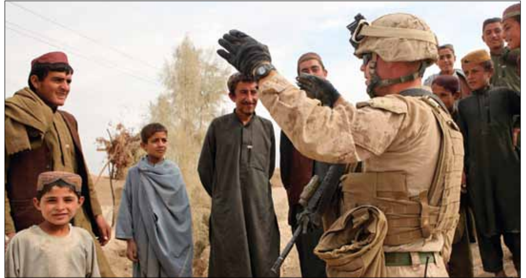
Chief Warrant Officer Brandon Smith speaks with residents while his unit conducts road repairs in Helmand province, Afghanistan, Nov. 3. Marines with 7th ESB repaired multiple areas along Route 611 in support of Operation Eastern Storm and after redeploying, 9th ESB continued to make progress on the major thoroughfare. Smith is the officer-in-charge of Heavy Equipment Platoon, Support Company, 7th Engineer Support Battalion, 2nd Marine Logistics Group (Forward). Photo by Cpl. Katherine M. Solano
